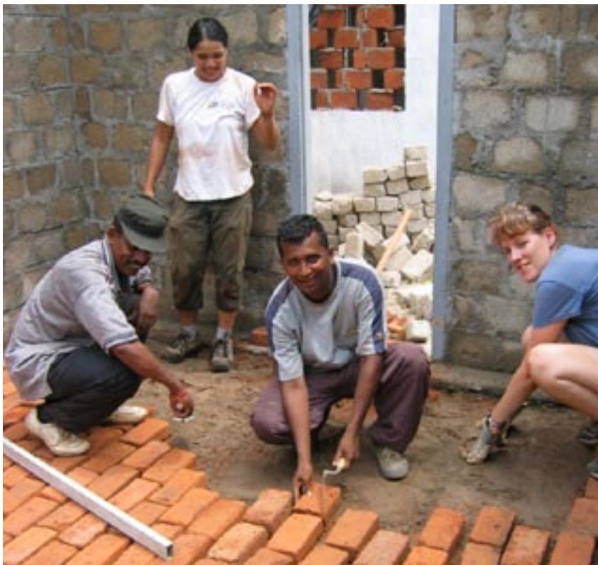
Building a brick floor in one of the new houses.
